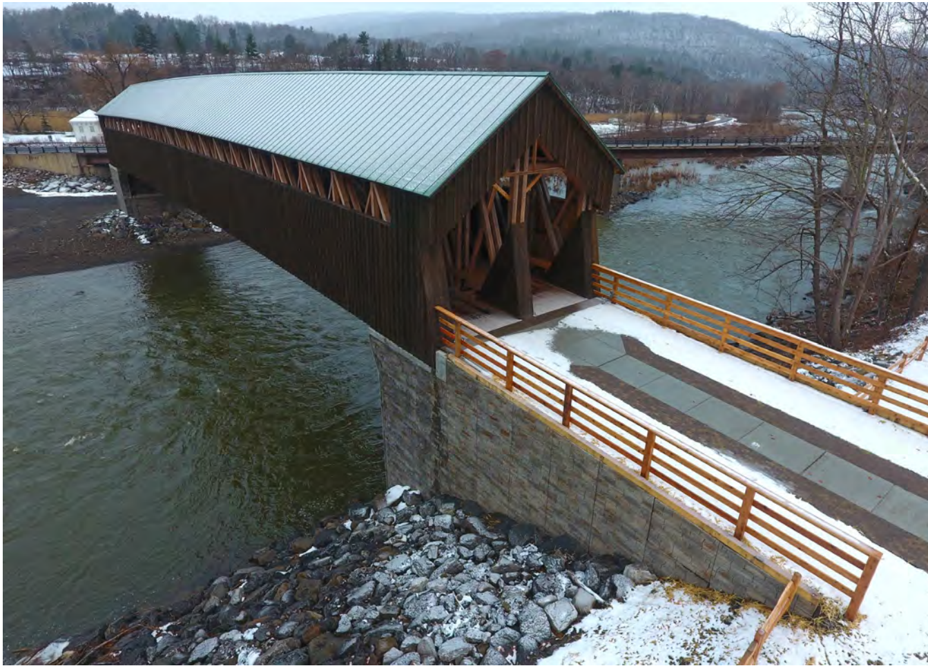
Completed Covered Bridge (East Side)
