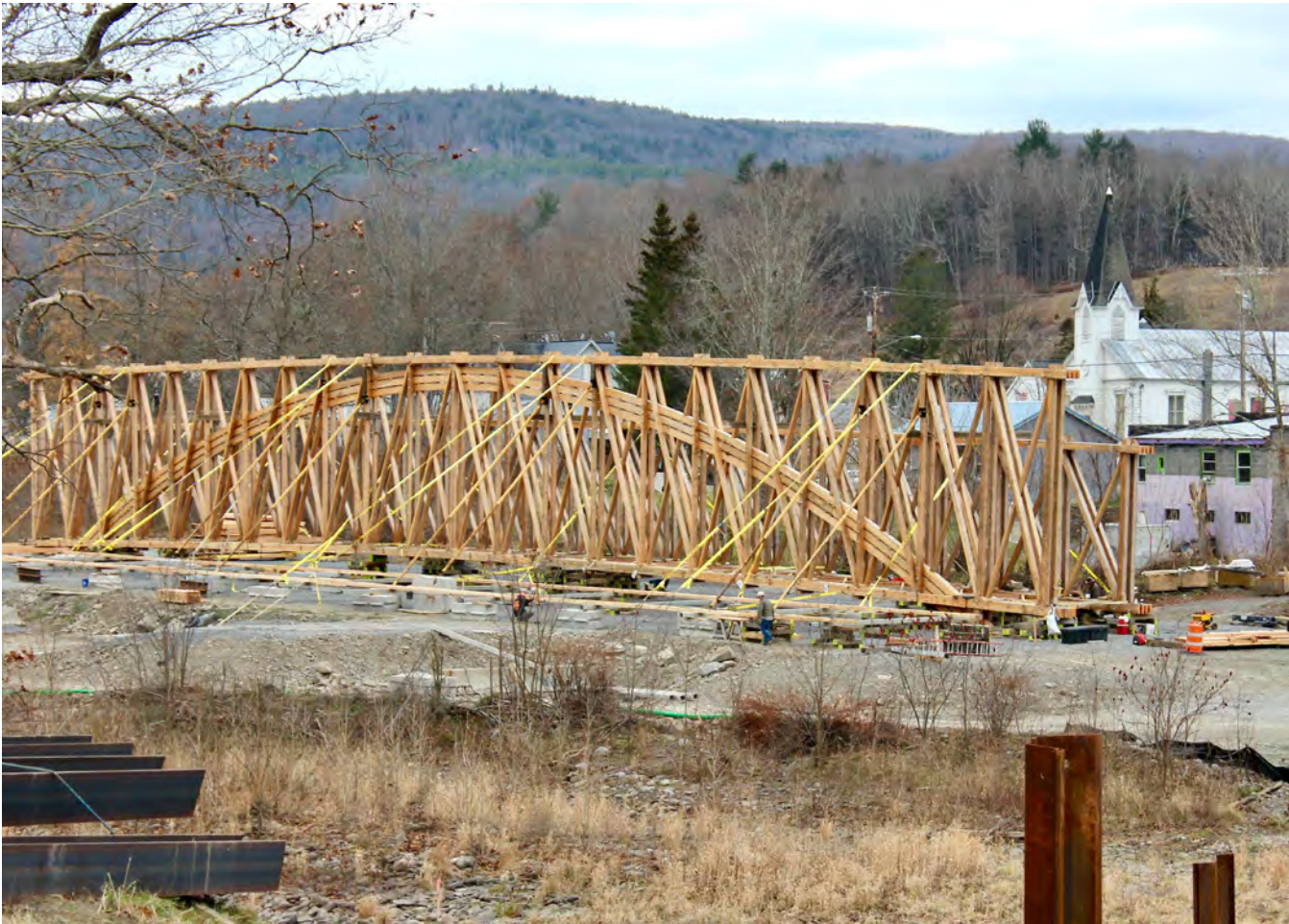
Economy Paving Co. employees two cranes to lift south truss
