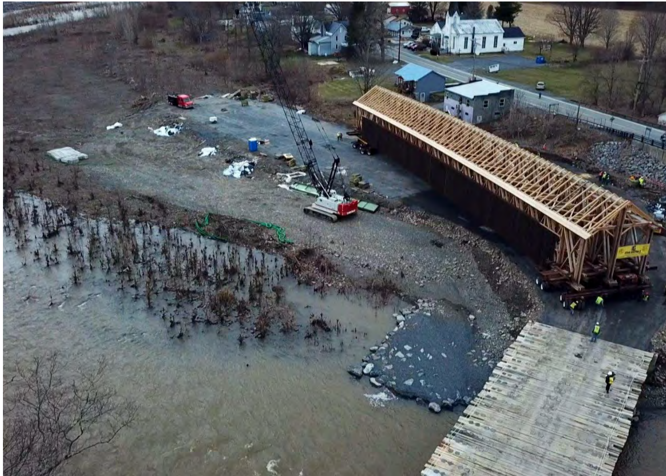
New covered bridge ready to slide onto temporary bridge
