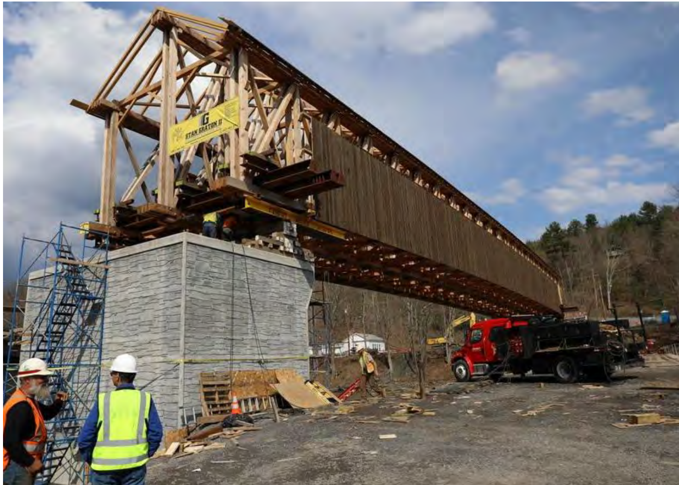
New covered bridge getting lowered onto the new abutments
