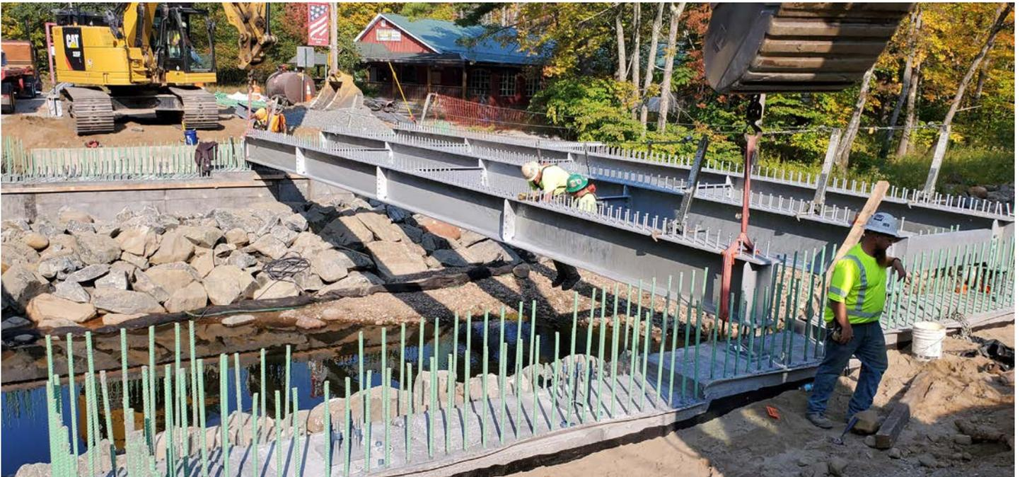
*Erecting Galvanized Steel Beam Superstructure*
