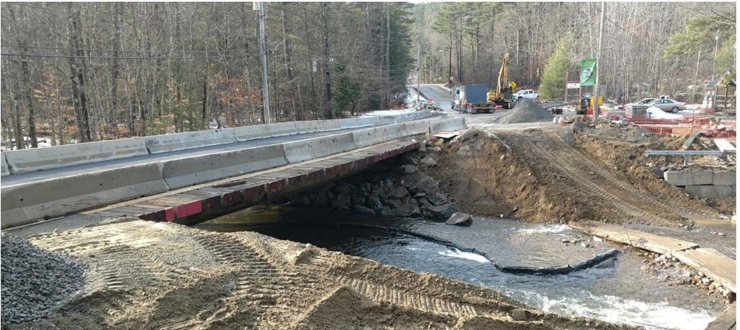
*Temporary 2-Lane Bridge Constructed on Adjacent Alignment to Accommodate Traffic During the Winter*
