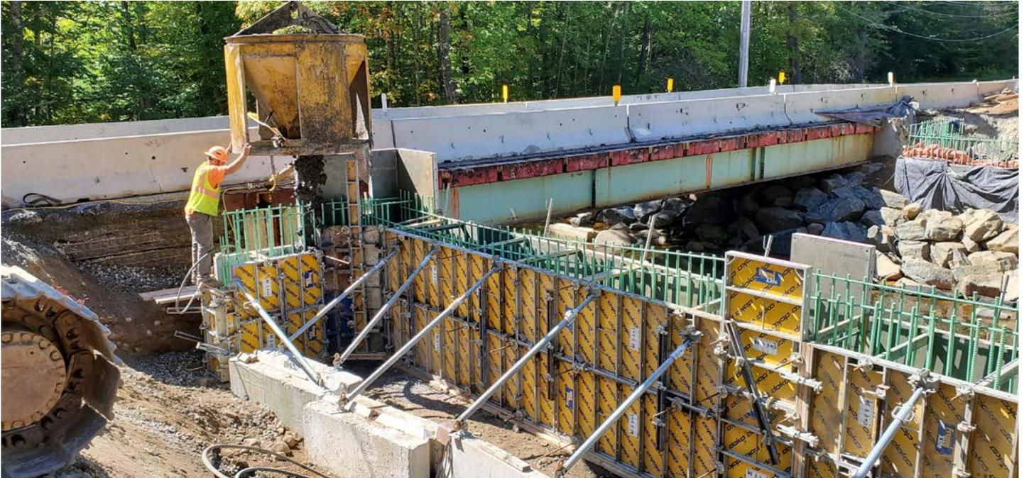
*Pouring Concrete for Integral Abutments*
