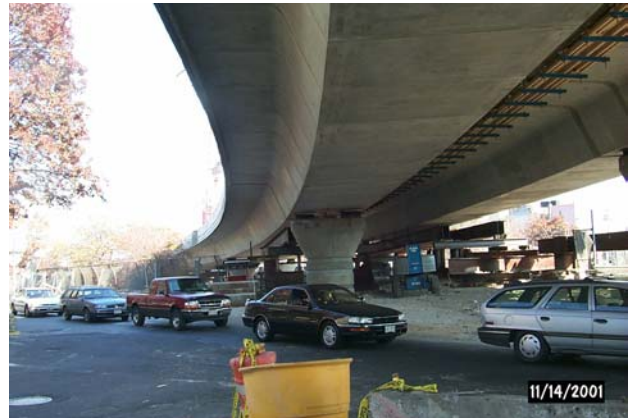
Figure 3 - Williamsburg Bridge Approach near completion using 3 meter long precast segmental units
