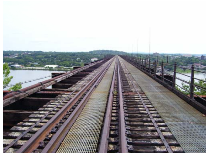
A current view of the bridge surface
