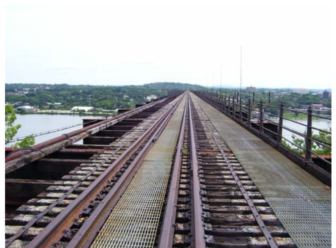
A current view of the bridge surface
